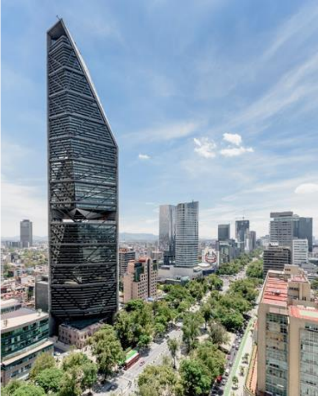
Torre Reforma, 2016, Foto © Moritz Bernouilly
