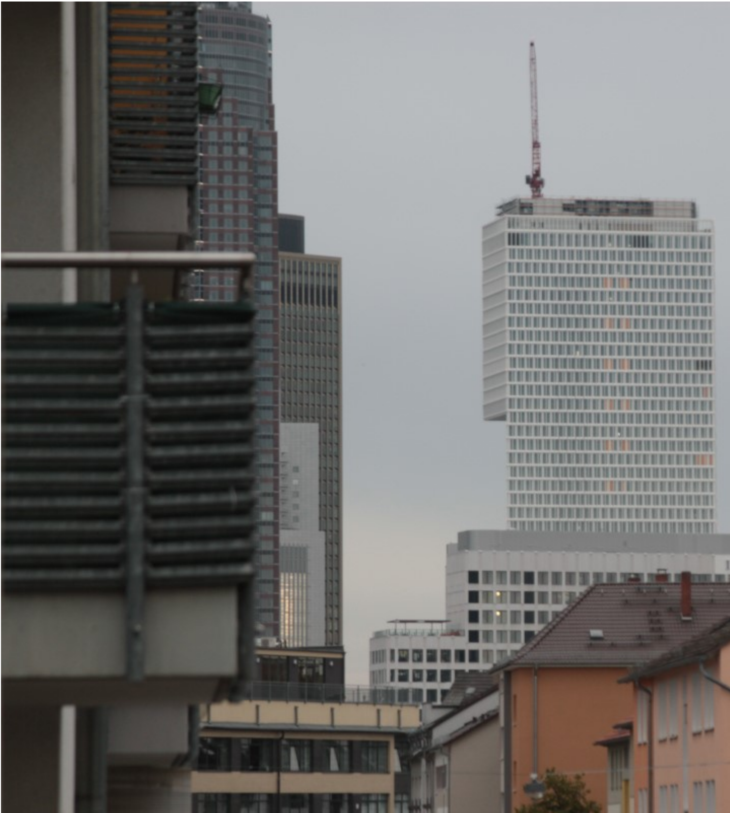
Bauphase Tower ONE, September 2021
