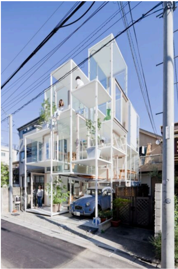
House NA, Tokio, Japan, 2011, Architektur: Sou Fujimoto Architects, Photo © Iwan Baan
