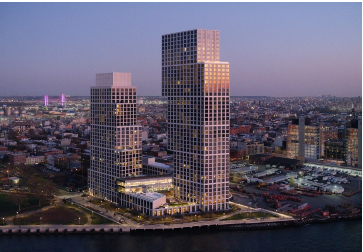
Eagle + West, New York, USA Architektur: Office for Metropolitan Architecture, Rotterdam, Niederlande
